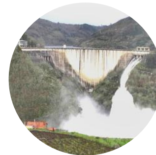
Hydroelectric Power Plants 1,138 MW
